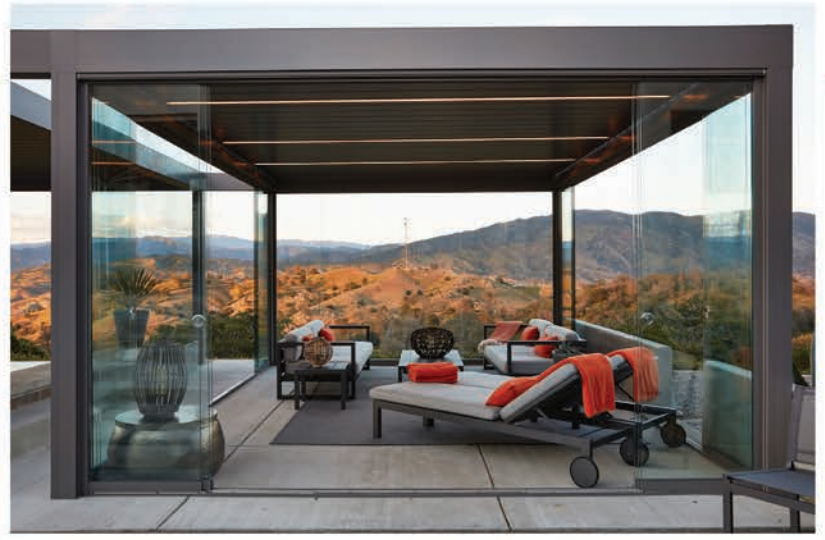
Photo Credits: 360 Aloft LLC Camargue structures shown with glass doors and shades.
